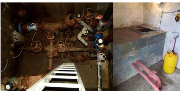
**Figure 4.** The fitting chamber of the tank with flowmeter (on the left), dosing of the disinfection and an open entrance to the water level in storage reservoir
