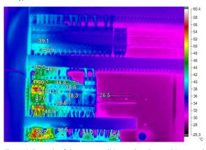
Figure 4. Example of thermogram (biogas plant 2 – machine room)
