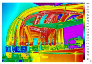
Figure 6. Example of thermogram (biogas plant 2 – transformer object)
