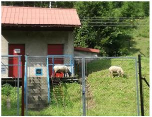
**Figure 1.** Corruption of the security barrier of the reservoir storage tank. In case of failure of the horizontal ceiling insulation of the tank, contamination of drinking water can result in faecal pollution.
