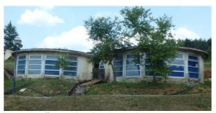
**Figure 3.** Insufficient technical condition and inappropriate construction of the water treatment plant. Large solar windows transmit the sunlight to the surface of the treated water, which promotes the growth of green algae in the treated water.
