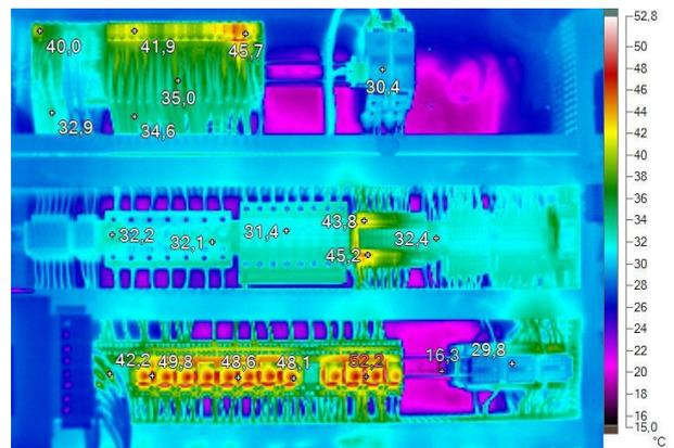
Figure 8. Example of thermogram (biogas plant 3 – control room)
