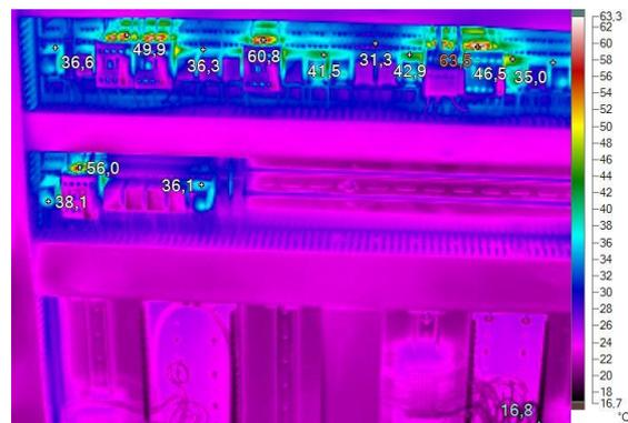
Figure 2. Example of thermogram (biogas plant 1 – control room)
