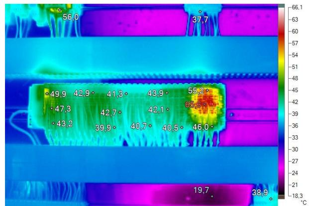
Figure 7. Example of thermogram (biogas plant 3 – machine room)
