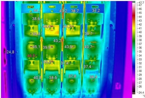
Figure 5.: Example of thermogram (biogas plant 2 – control room)
