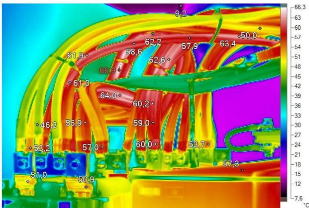
Figure 6. Example of thermogram (biogas plant 2 – transformer object)
