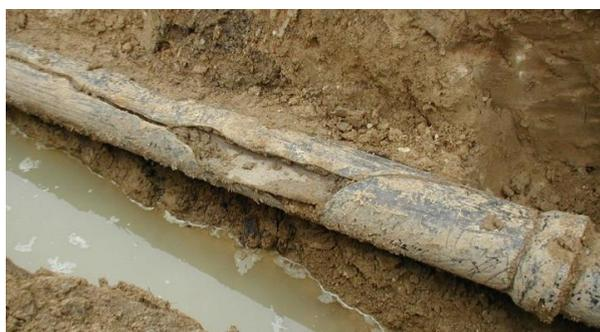
**Figure 2.** Safety barrier violation of the water distribution network. Insufficient technical condition of the pipeline. When pressure drops in the water supply network, penetration of environmental pollution into the water pipe may occur.
