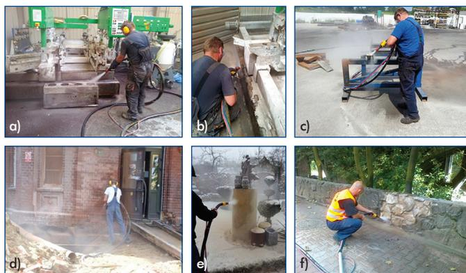
Fig. 2. Examples of using the Sandbot device: a), b), bodies of machines renovation; c) descaling and cleaning of welds; d), e), f) building surface renovation
